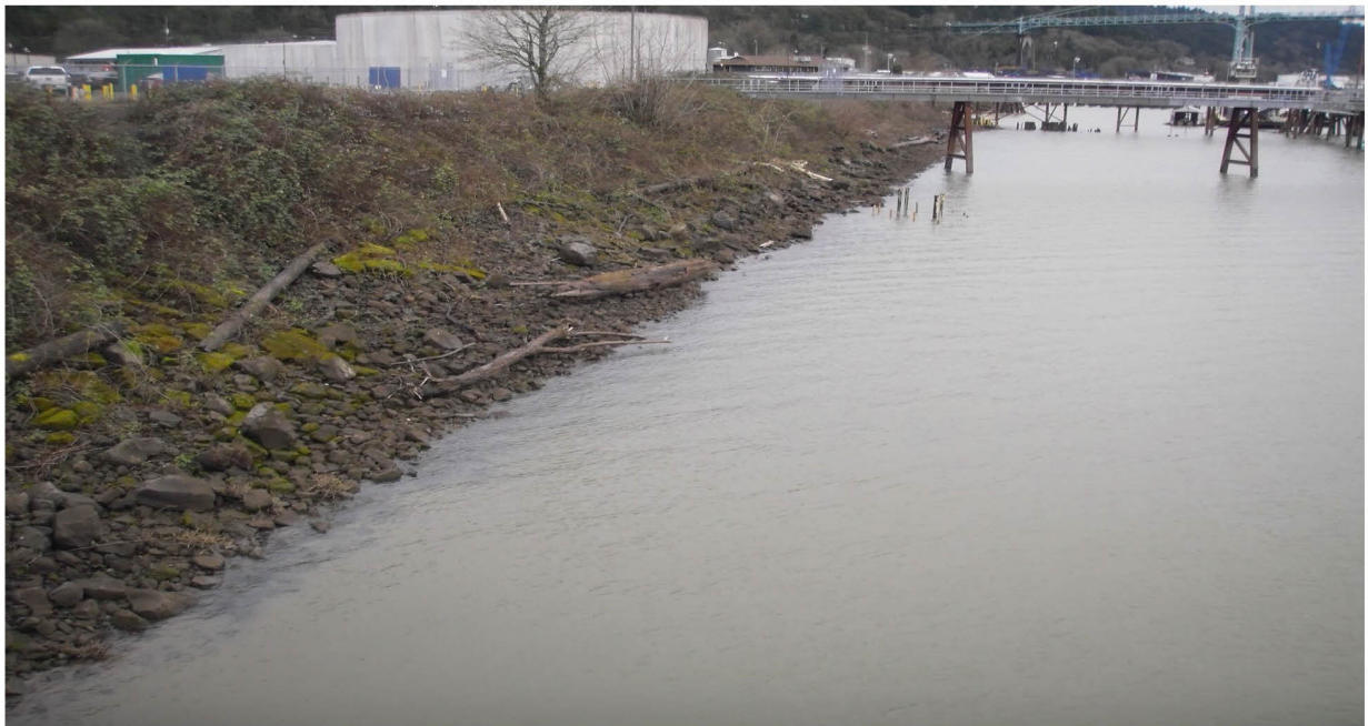
Photo 2 River Level Currently Above the Extent of Sediment Cap (1/22/2020)
