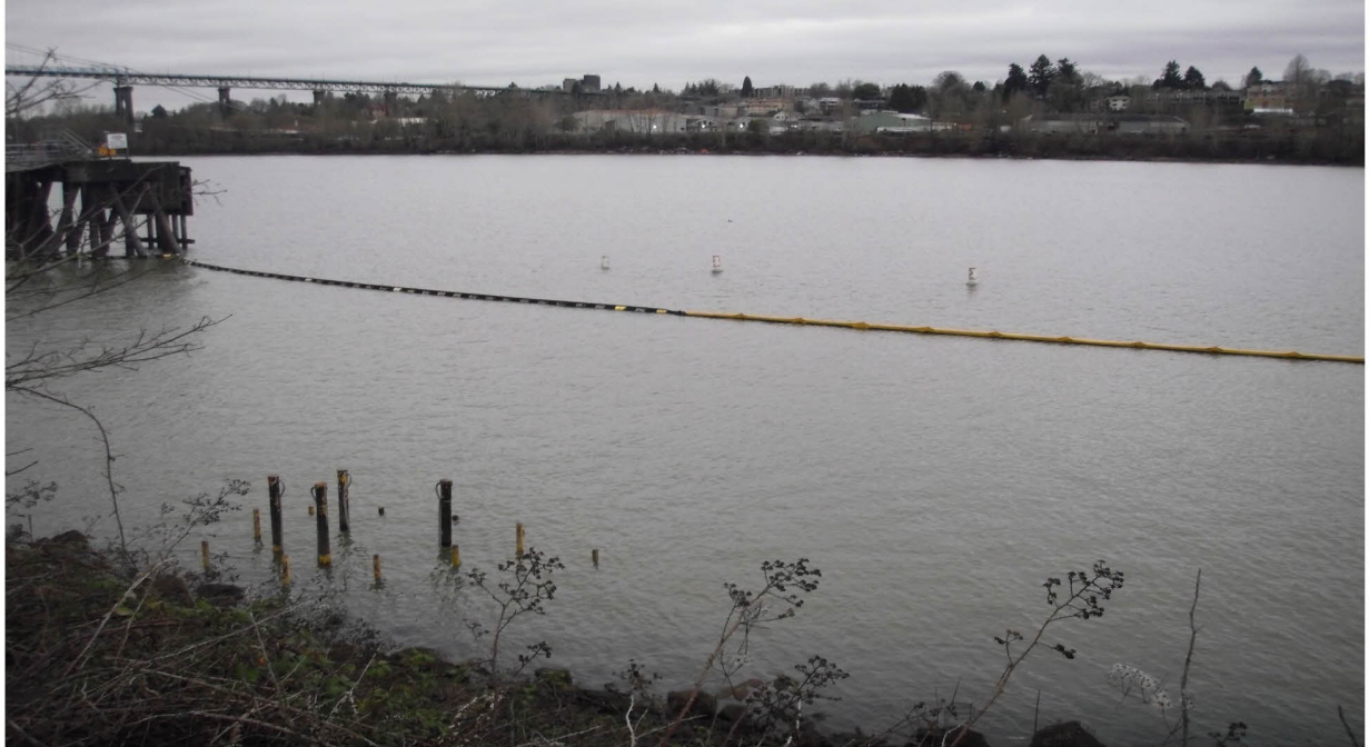
Photo 1 PacTerm Oil Boom Placement from Dock to Dolphin with Three Mariner Warning Buoys at Pilot Cap Area (1/22/2020)
