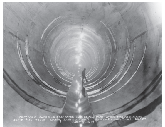
A worker inspects 22-foot-diameter "pressure tunnel" that will feed water to Lower Baker Dam powerhouse. (October 1925)
