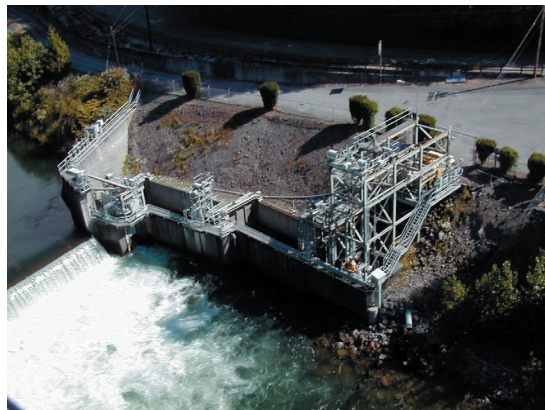
Migrating salmon are trapped in this facility below Lower Baker Dam and then are trucked upstream for release above Upper Baker Dam.
