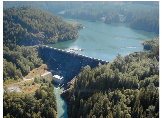
Upper Baker Dam
