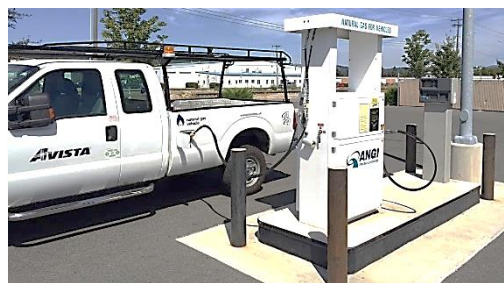
Above: Compressed Natural Gas station at Mission Campus Left: Avista natural gas-powered work truck
