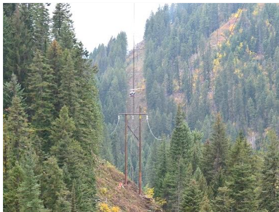
Above: Some of the terrain Avista line crews face (Pine Creek – Burke Thompson line)
