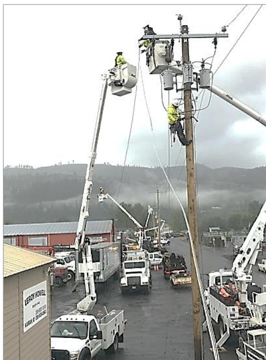
Using a variety of different sizes of bucket trucks and support vehicles to repair storm damage in Kamiah
