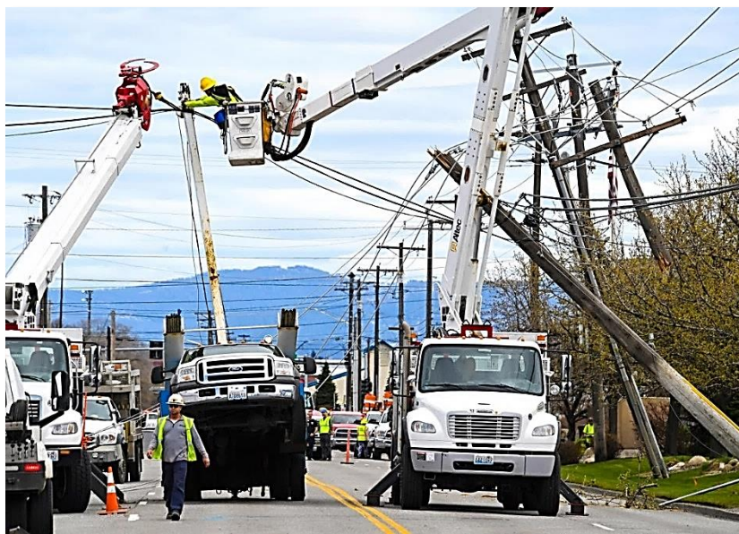
Avista crews work to free a customer vehicle that snagged distribution lines. They use a digger derrick (left) to hold the lines up and a bucket truck (right) to place the lineman into position.
