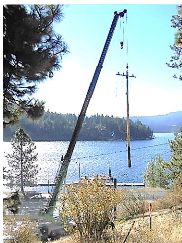
Left: Crane setting a pole on a steep hillside.
