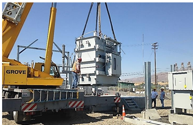
Work on the Lee & Reynolds Substation in 2018
