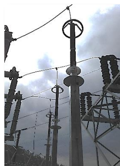
Lightning arresters at Lakeview Substation
