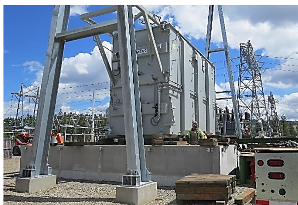
New Westside #1 230/115 kV transformer being put into place
