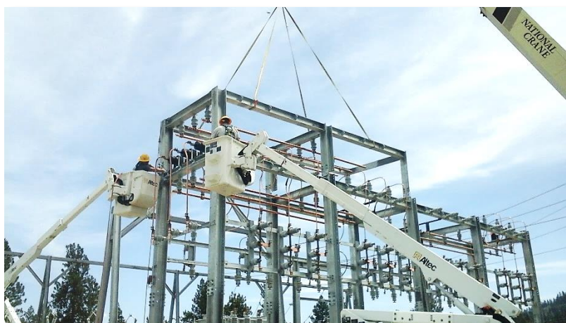
Work on the Ninth & Central Substation
