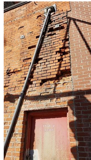
Post Street Substation Wall
