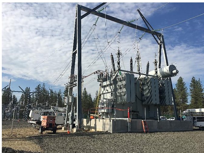
Installation of new autotransformer at Westside Sub
