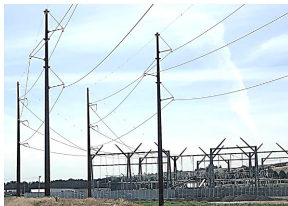
Saddle Mountain Substation under construction
