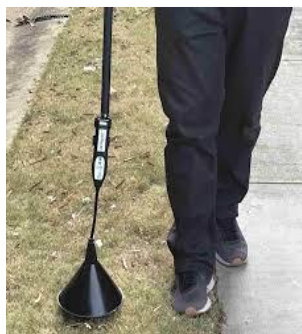
Pipeline Leak Detection
