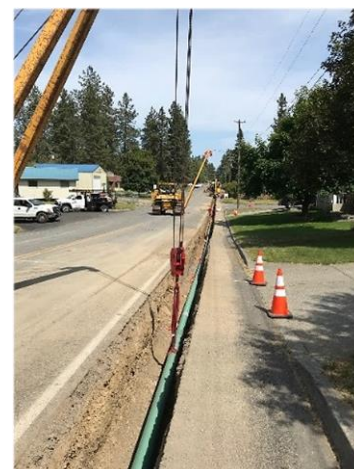
Gas Line Relocated for Road Work
