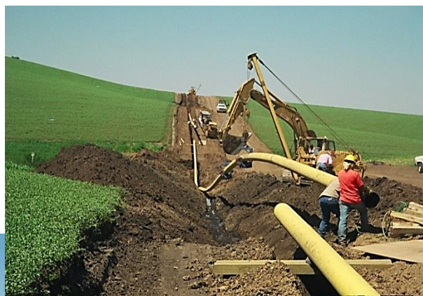
Installing natural gas pipeline across the Palouse
