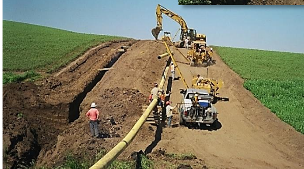
Installing natural gas pipeline across the Palouse
