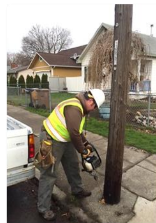
Avista Wood Pole Inspection
