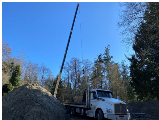
(Above) Construction is underway for the new reservoir
