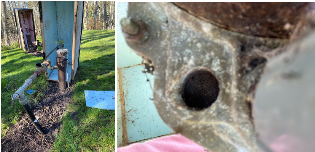
(L) Well #1 with sample tap and source meter (R) Screened vent on Well #1
