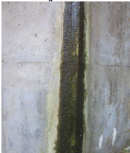
Leaking reservoir corner
