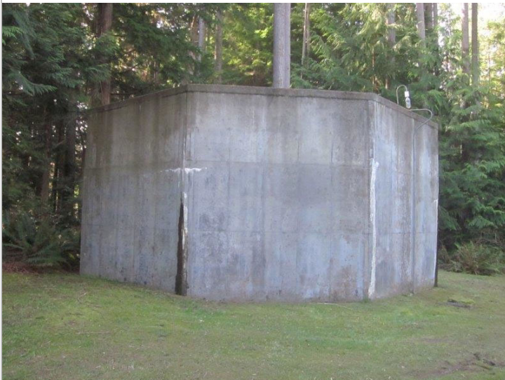
Leaking reservoir corner
