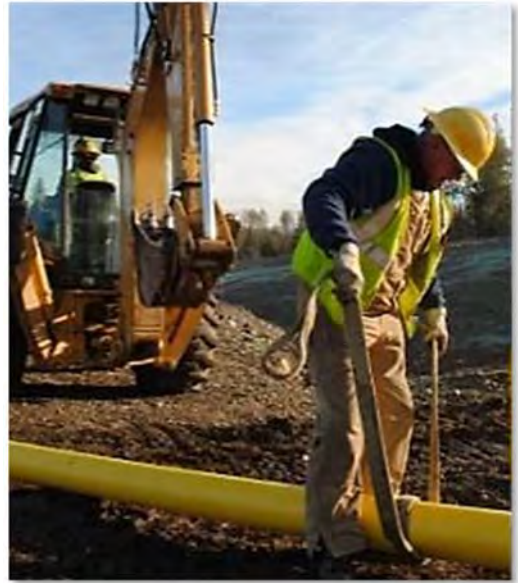
Figure 8. Natural Gas Pipe Installation
