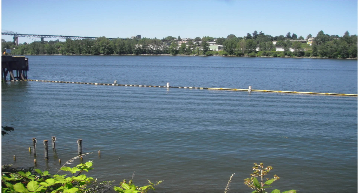
Photo 1 PacTerm Oil Boom Placement from Dock to Dolphin with Three Mariner Warning Buoys at Pilot Cap Area (6/26/2020)
