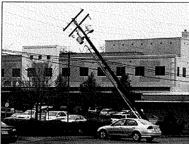
Linnette Engler sent in this photo of wind-blown power lines in Bellingham
