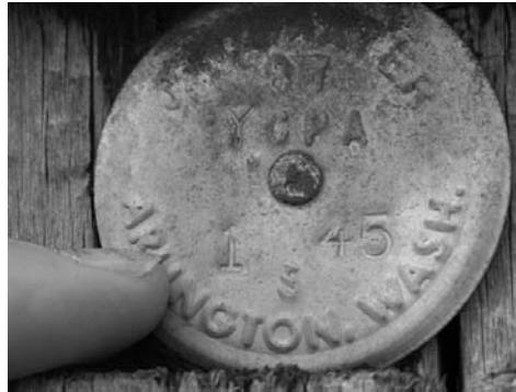
Figure 1 Typical Pole Tag in Pole Gain
