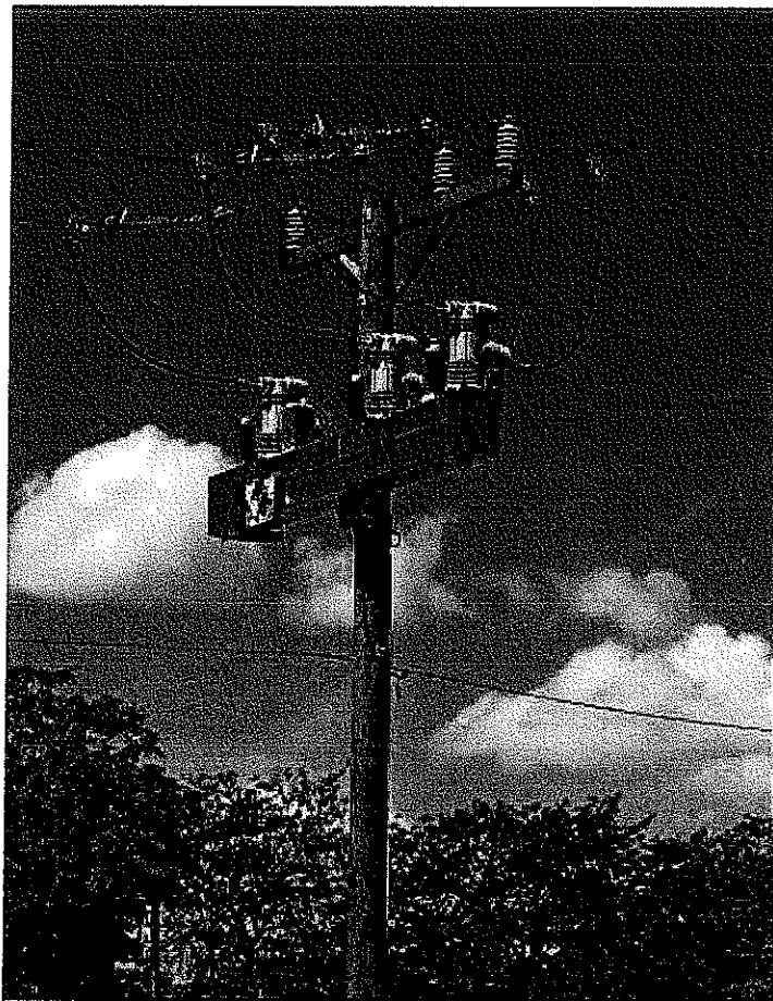
Figure A5. Hi-Tech Automation Switch
