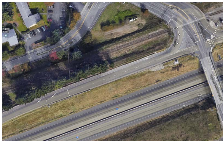
Figure 2. Barksdale Avenue Satellite View
