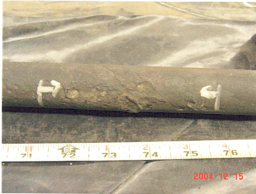
Figure 5. Photograph of Segment 2 showing scratches in the coating between the 71-inch and 75.5-inch locations with a dent in the coating at the 73.5-inch location.
