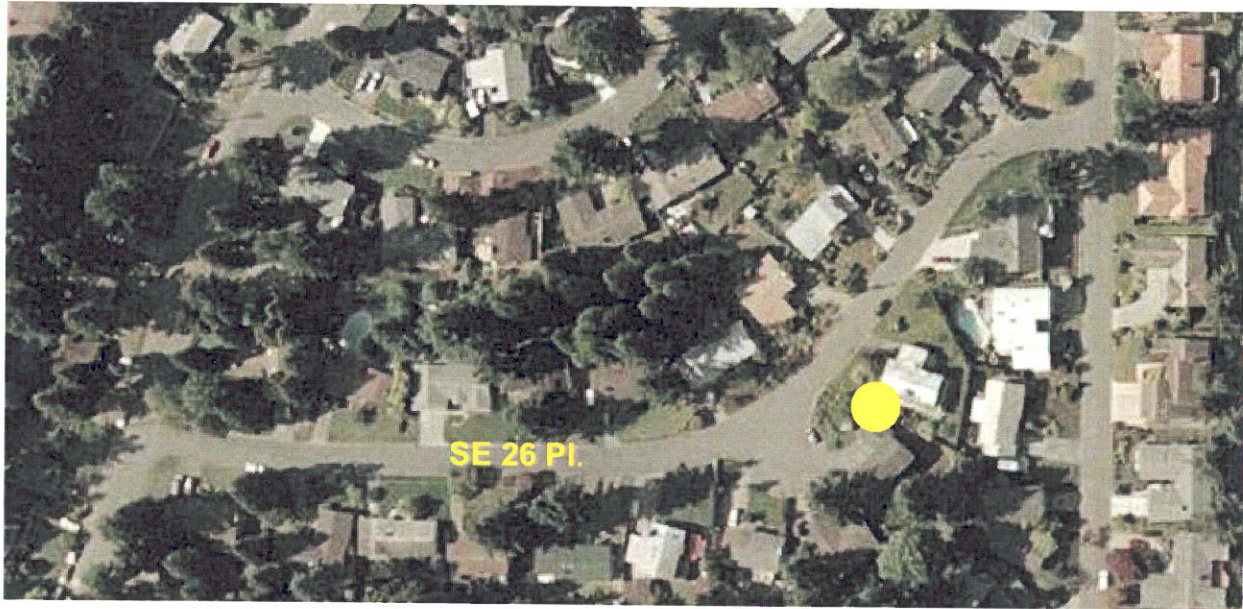
Figure 1. Aerial view of the failure site location in Bellevue, WA (taken in 2002).
