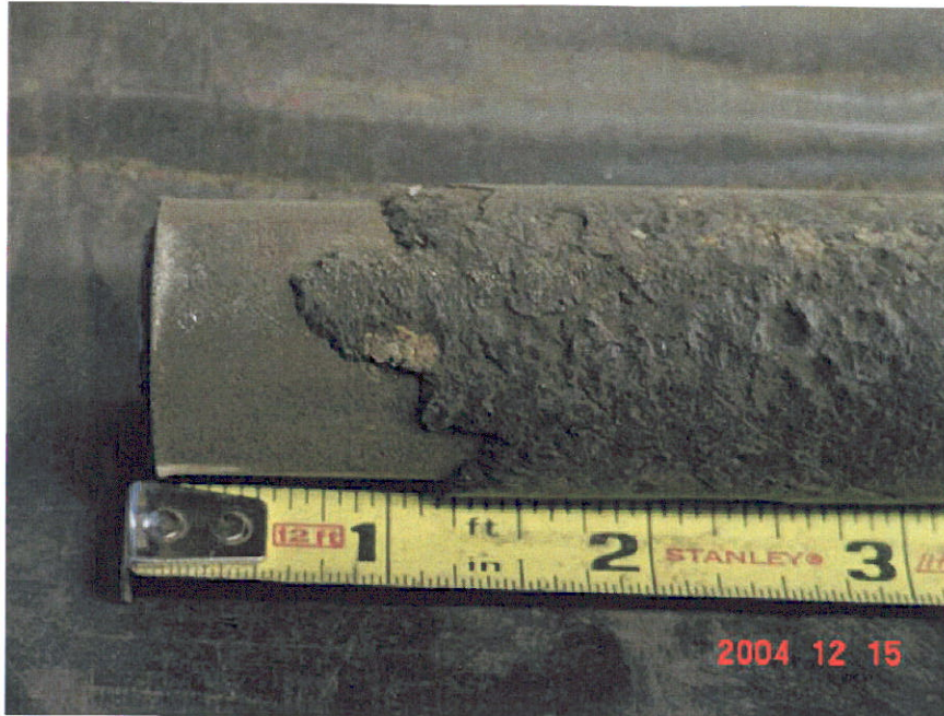
Figure 7. Photograph of Segment 4 showing an area of bare pipe between the 0-inch and 1.5-inch locations.
