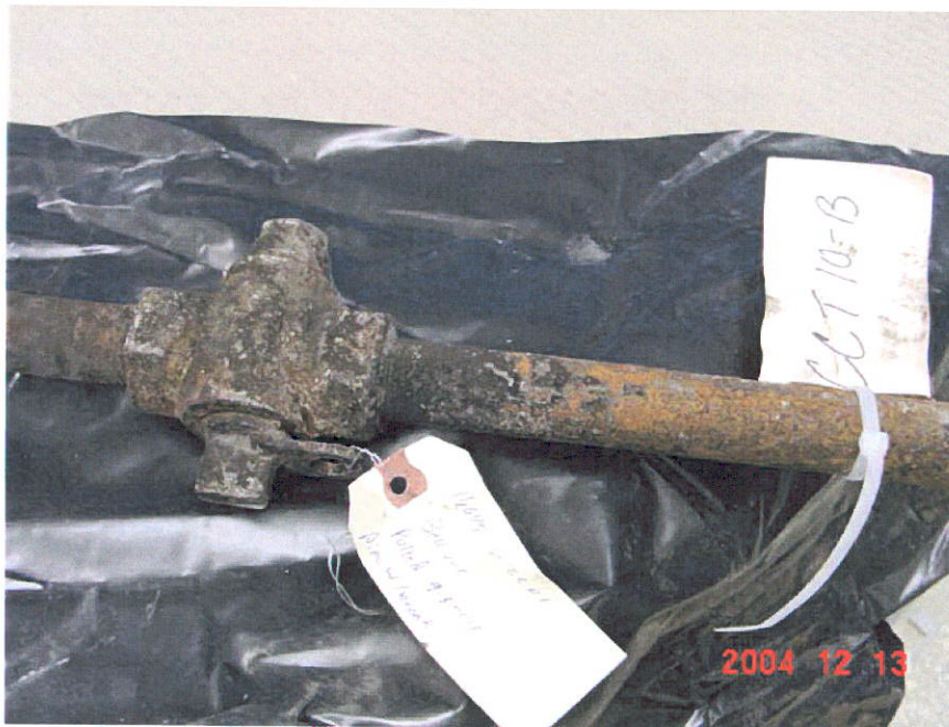
Figure 38. Photograph of unwrapped Segment 10 showing a valve on the downstream side of the pipe, CCT 10-B.
