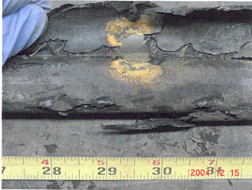
Figure 11. Photograph of Segment 9 after a portion of the coating was removed revealing an anomaly at the 29.5-inch location.
