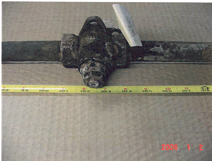
Figure 38. Photograph of Segment 10 showing the valve that was located at the 102.5 inch location.
