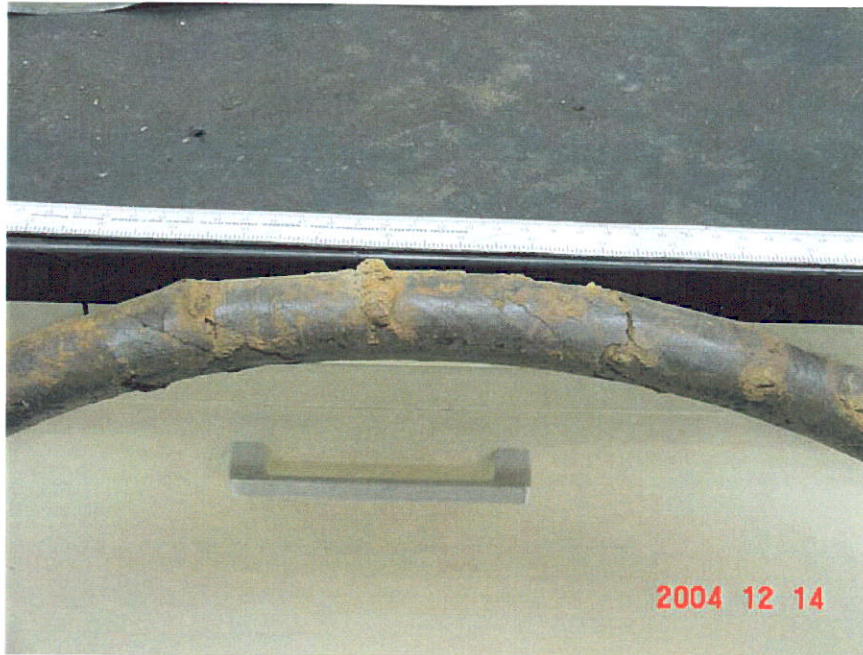
Figure 35. Photograph of Segment 10 showing the nodules that were in coating deformations on the extrados of the pipe.
