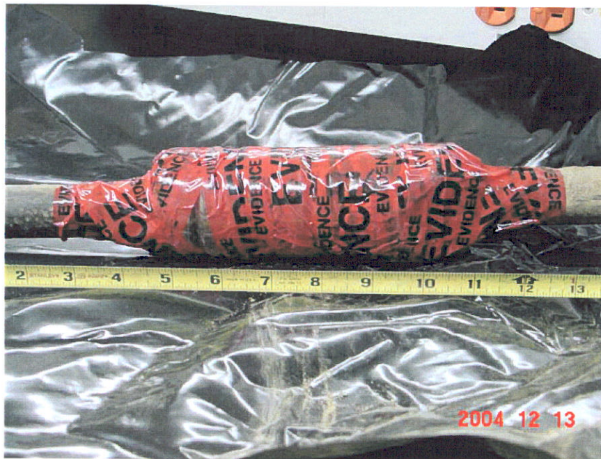
Figure 36. Photograph of unwrapped Segment 10 showing red evidence tape on a protective covering on the pipe.
