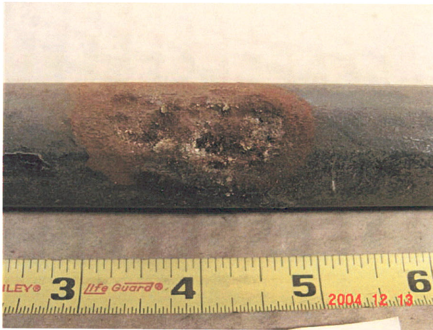
Figure 4. Photograph close-up of Segment 1 after removal of protective wrapping for shipping.
