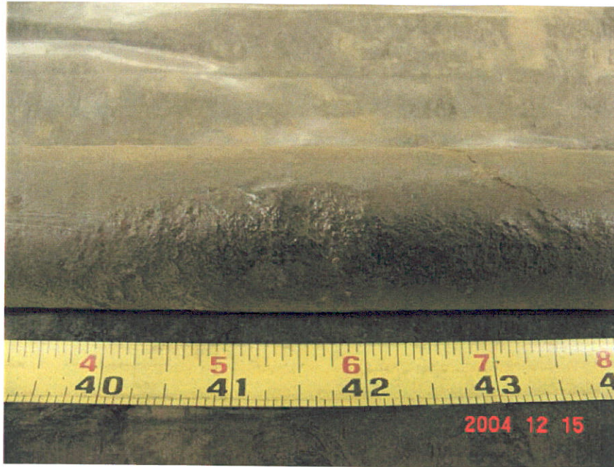
Figure 13. Photograph of Segment 6 showing a dent in the coating at the 41.5-inch location.
