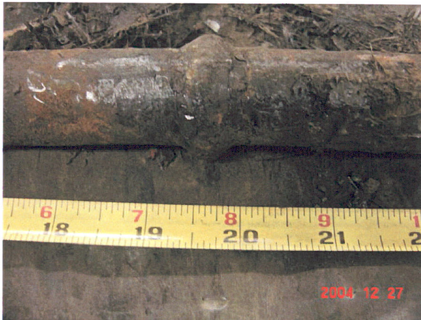
Figure 10. Photograph of Segment 8 after the coating wrap and coating was removed revealing a weld at the 19.5-inch location.
