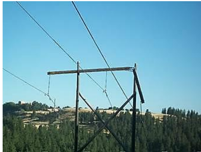
Examples of damaged crossarms
