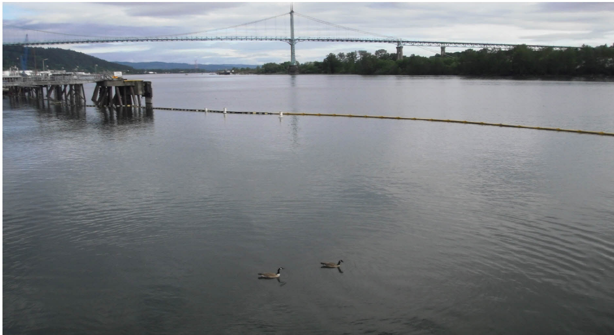
Photo 1 PacTerm Oil Boom Placement from Dock to Dolphin with Three Mariner Warning Buoys at Pilot Cap Area (5/21/2020)
