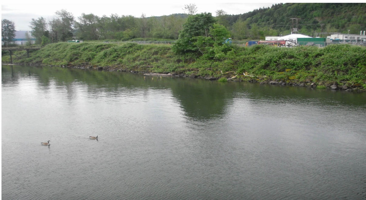
Photo 2 Mat Material Not Visible Due to High River Water Elevation (5/21/2020)
