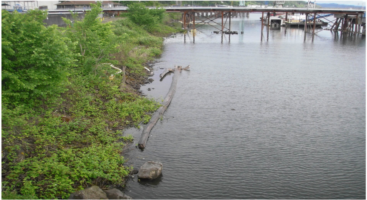
Photo 3 Conditions Immediately Downriver of Cap Area (5/21/2020)
