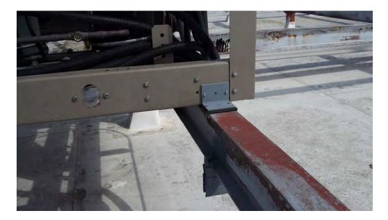
Photo 17: Minimal Equipment Connection
