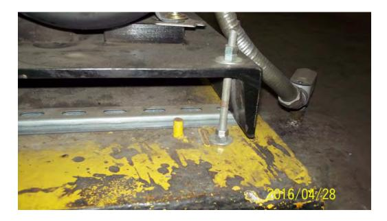
Photo 19: No apparent Lateral Connection of Pump to Base
