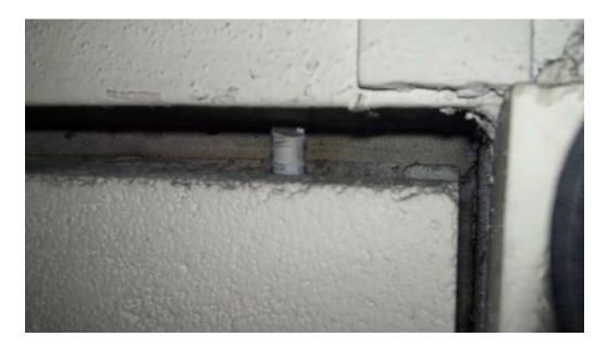
Photo 6: Concrete Spandrel to CMU Wall Interface (Note: Lack of connection between the masonry below and the ledger angle above.)
