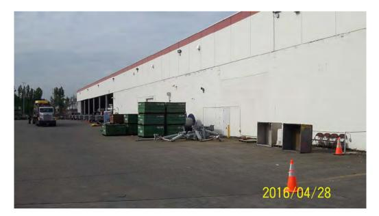
Photo 4: East Exterior Elevation – High Bay Warehouse (Note: Infill masonry wall below concrete spandrel.)
