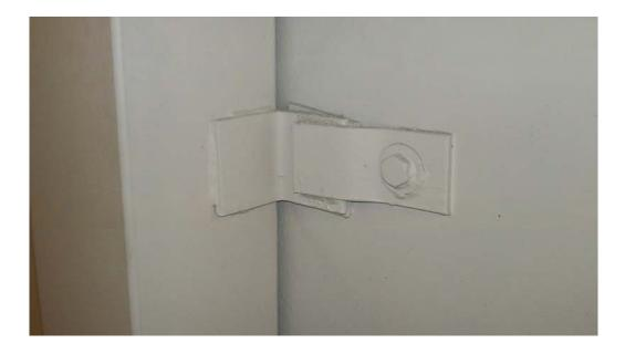
Photo 12: Concrete Wall to Column Clip
