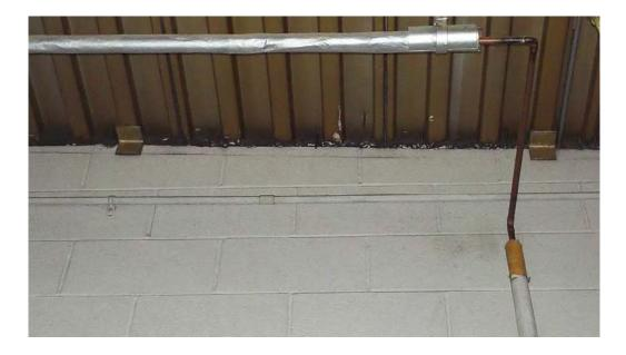
Photo 14: Minimal Clips at Top of Masonry Partition Walls
