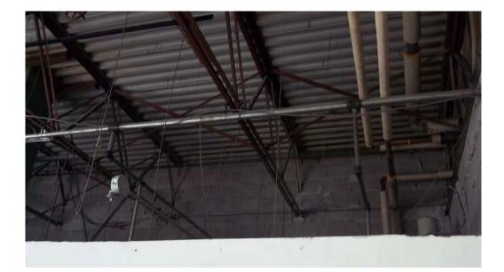
Photo 15: Masonry Partition Framed Around Joist (Note: How the Masonry is grouted around the Joist, potentially overstressing the Joist.)
