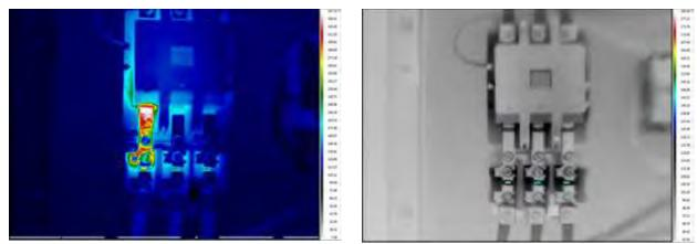
This heat signature suggests that an issue lies in the internal components of the contactor.
