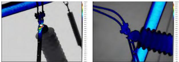
The heating on this outdoor utility switch is likely caused by resistance from a corroded or loose connection.
