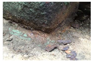
The fuel yard is subject to a very corrosive environment due to the wet wood being in contact with the equipment. The years of rusting has caused failure to metal conduit and structural steel. The metal support structure of the truck receiving hoppers has rusted through to the point of being completely cracked through. Welded plates have been installed to affected areas on the truck receiving dumpers. Many of the electrical conduits are rusted through and need replacement.
