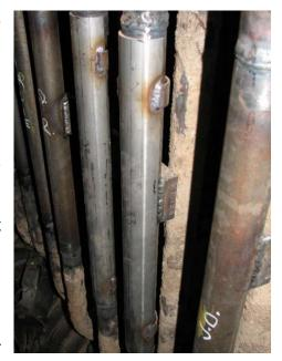
40% were discovered during scheduled outages. The secondary superheater has operated longer than expected and has thinning throughout the entire pendant. Data shows ongoing maintenance of sections will no longer be a viable option as much of the pendant has reached the Pink measurement.
