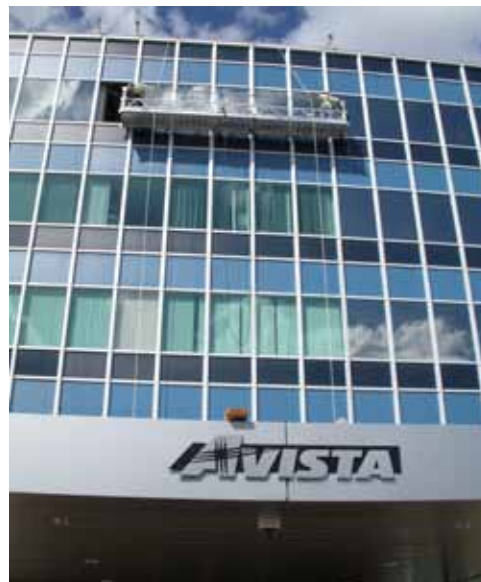
Energy efficient window replacement at Avista's headquarters in Spokane, Washington
