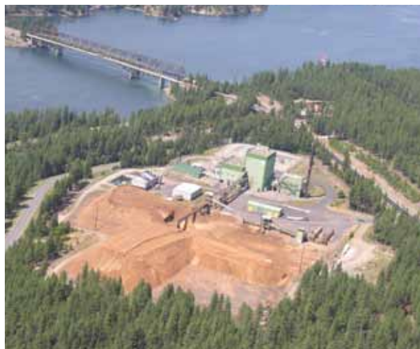
Kettle Falls Generation Station
