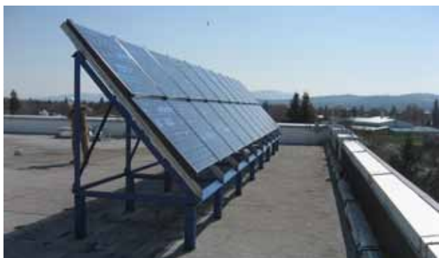
Newly installed solar panels at Avista's headquarters in Spokane, Washington
