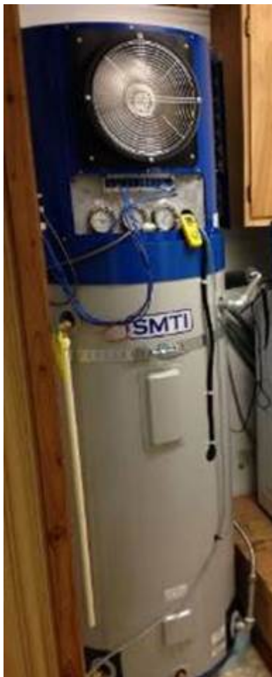
Figure 2.20: SMTI High Efficiency Heat Pump Water Heater 48
