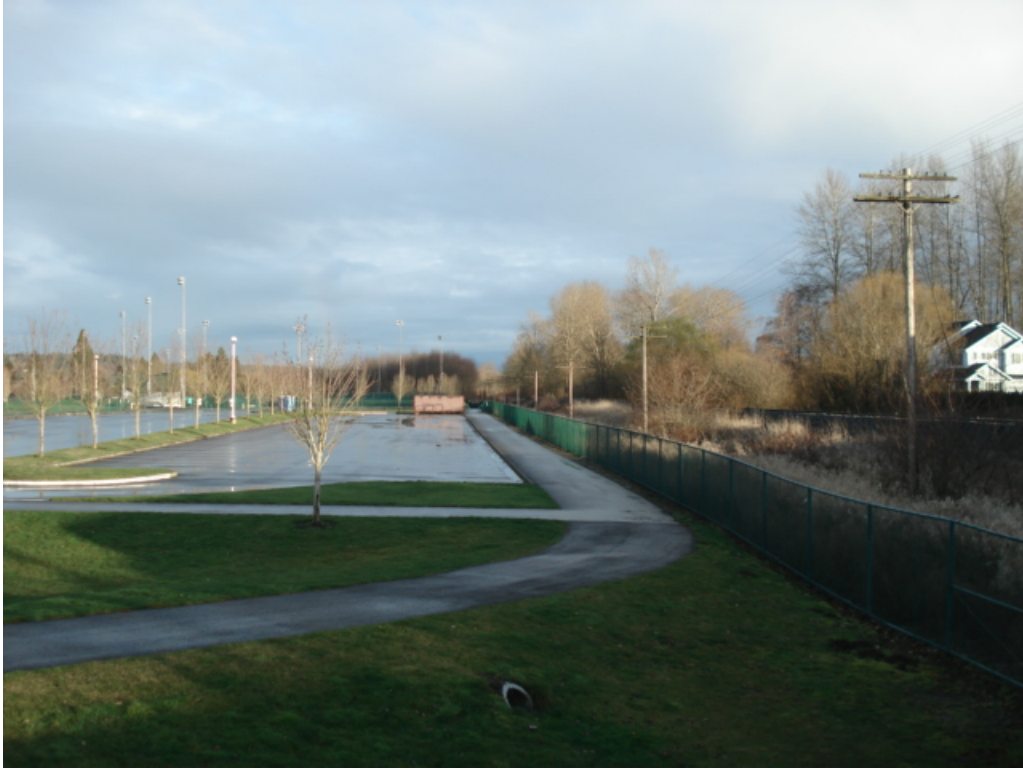
Figure 3 20' North of Crossing Right-of-Way/Fence Looking East
