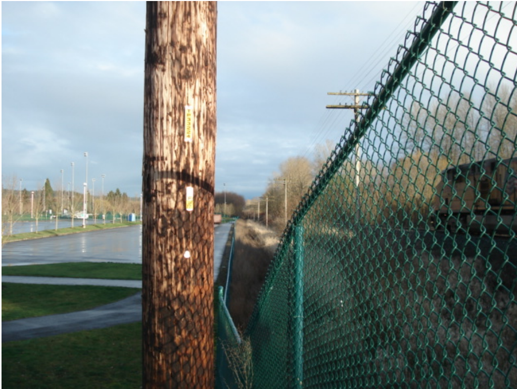
Figure 2 North of Crossing at Right-of-Way/Fence – Looking East
