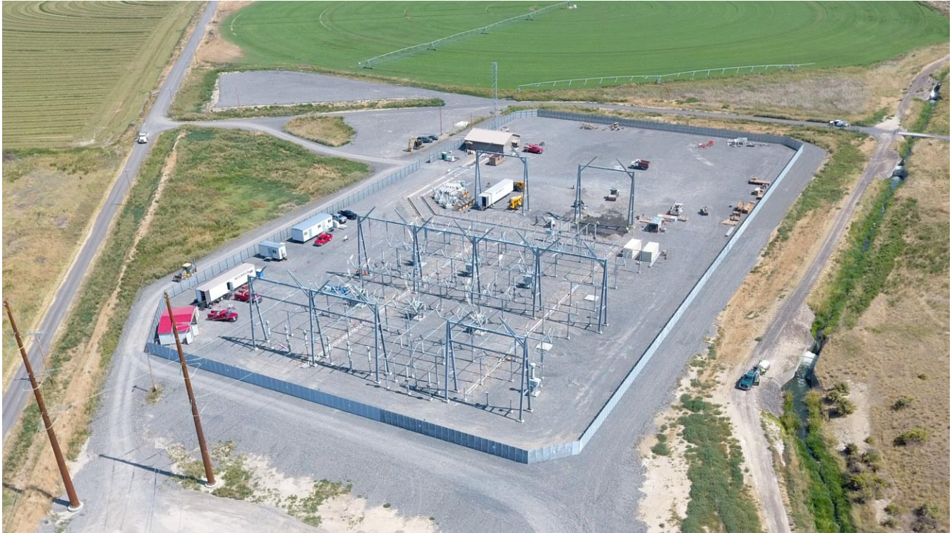
SADDLE MOUNTAIN STATION UNDER CONSTRUCTION
