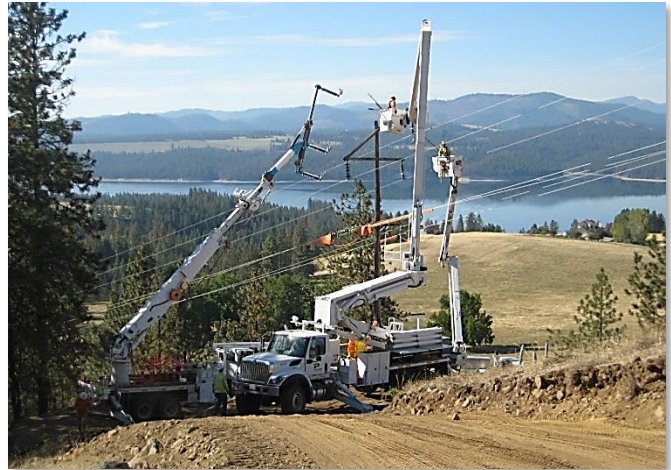
Figure 29. Addy-Gifford Steel Pole Replacement Work
