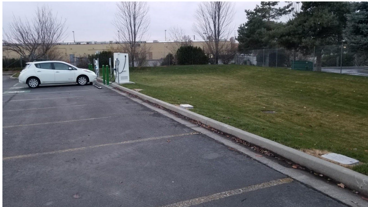
Liberty Lake STA park and ride, site ready for additional Level 1 Chargers?
