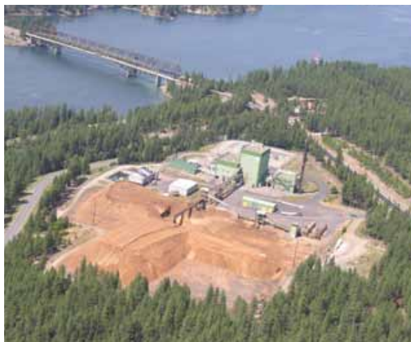
Kettle Falls Generation Station
