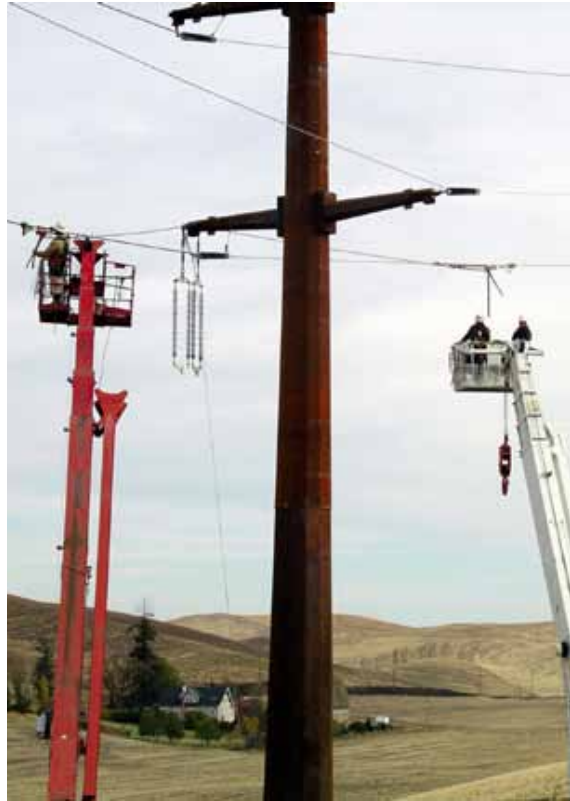
Transmission upgrade work
