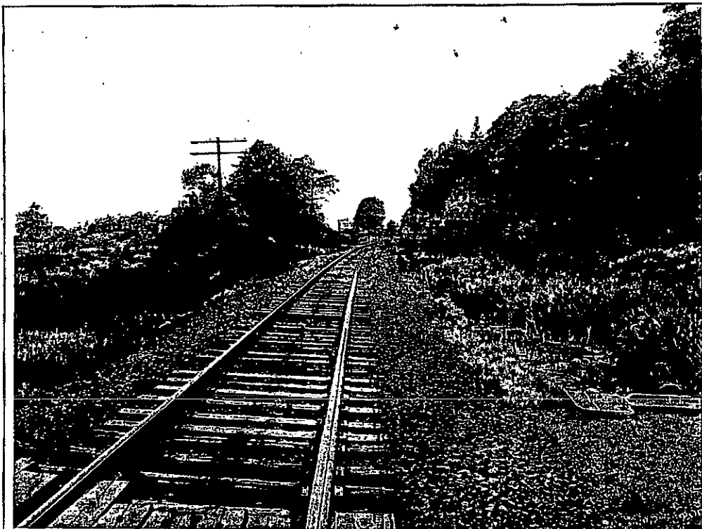
Photo 1: View looking north at intersection with Logen Road.
