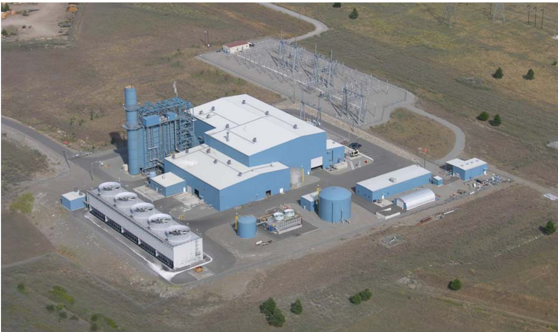
Lancaster Generation Facility
