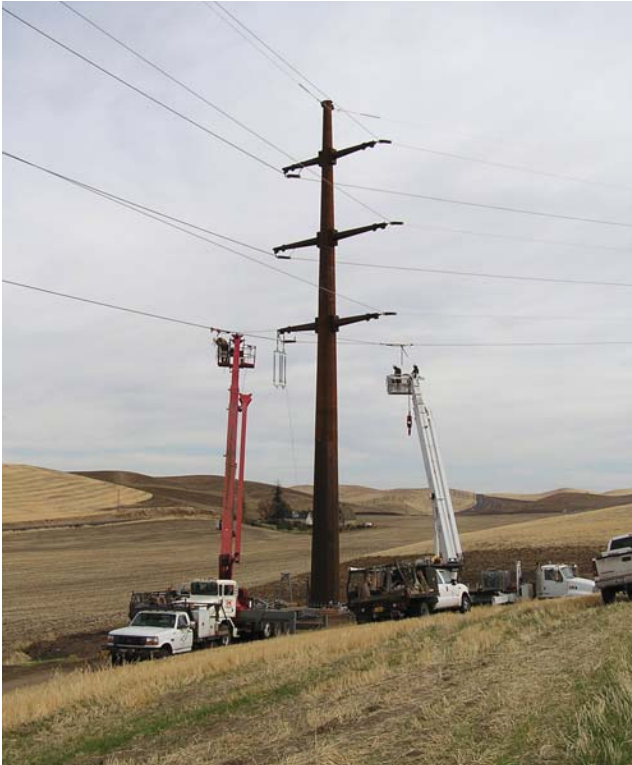
Transmission Construction in the Palouse Region, Southeastern Washington
