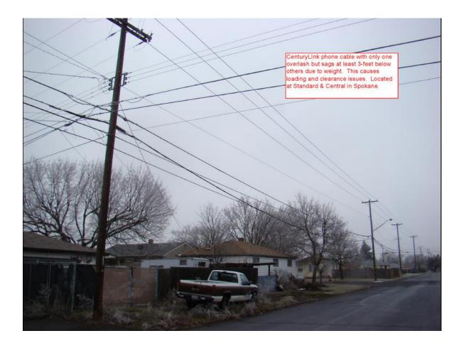
The process of evaluating proposed overlashing takes far longer than the seven days specified in Draft Rule 480-54-030(11). In order to manage safely the limited space on poles for the benefit of all, it is very important that main line cable overlashing require a Route Application and design prior to construction in the same manner as new wireline construction.
