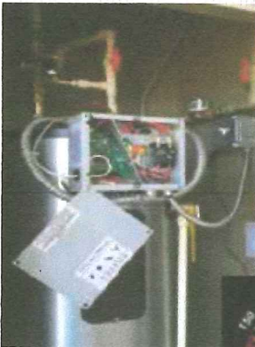
Left: GIWH control unit, installed on an electric water heater.
