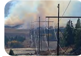
Operations & Emergency Response
