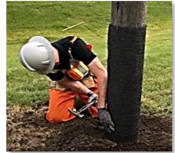
Installing Pole Wraps
