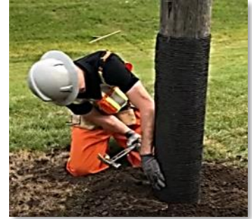
Installing Pole Wraps
