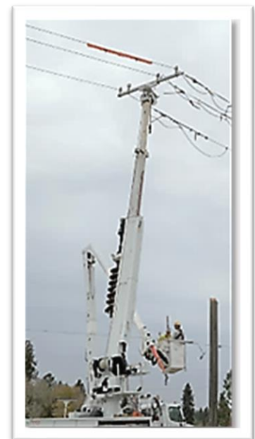
Figure 13. Grid Hardening Work
