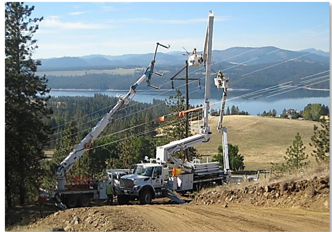
Figure 29. Addy-Gifford Steel Pole Replacement Work
