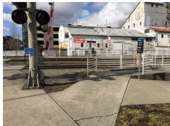
Looking west from north side
