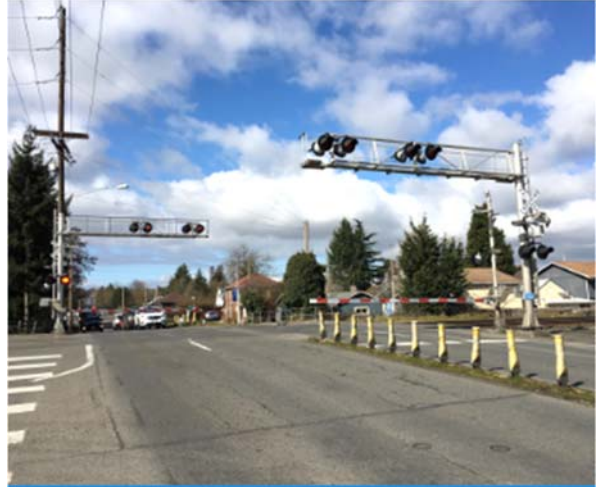
Looking west from south side.
