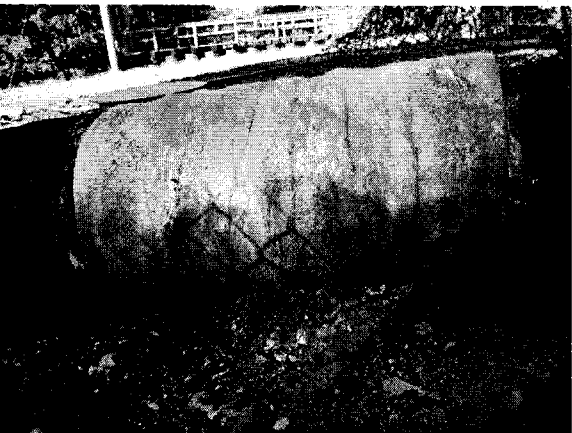
Figure 3. NE 11 th Avenue and NE Division water crossing, Camas, Washington: Close-up view of repair to pipe coating at point where concrete supports were removed.
