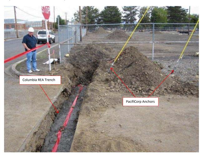
Example of Locate at Canberra: Locate performed by Columbia REA shows "No CREA". Locate performed by Locate Inc. shows that there are PacifiCorp facilities present.
