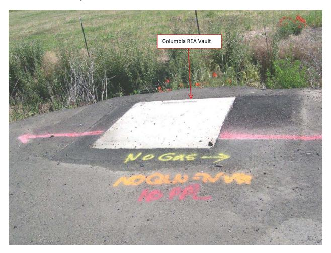
Columbia REA's proposed underground line does not meet PacifiCorp's six foot minimum clearance for separation of facilities. Columbia REA's proposed primary underground line is staked to run between PacifiCorp's pole and guy wire.
