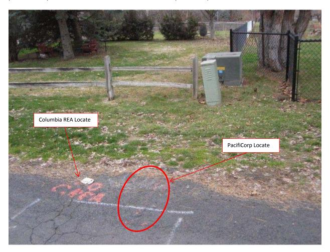
Example of Locate at Cottonwood: Locate performed by Locate Inc. indicates "No PPL". However, there is a Columbia REA vault present.
