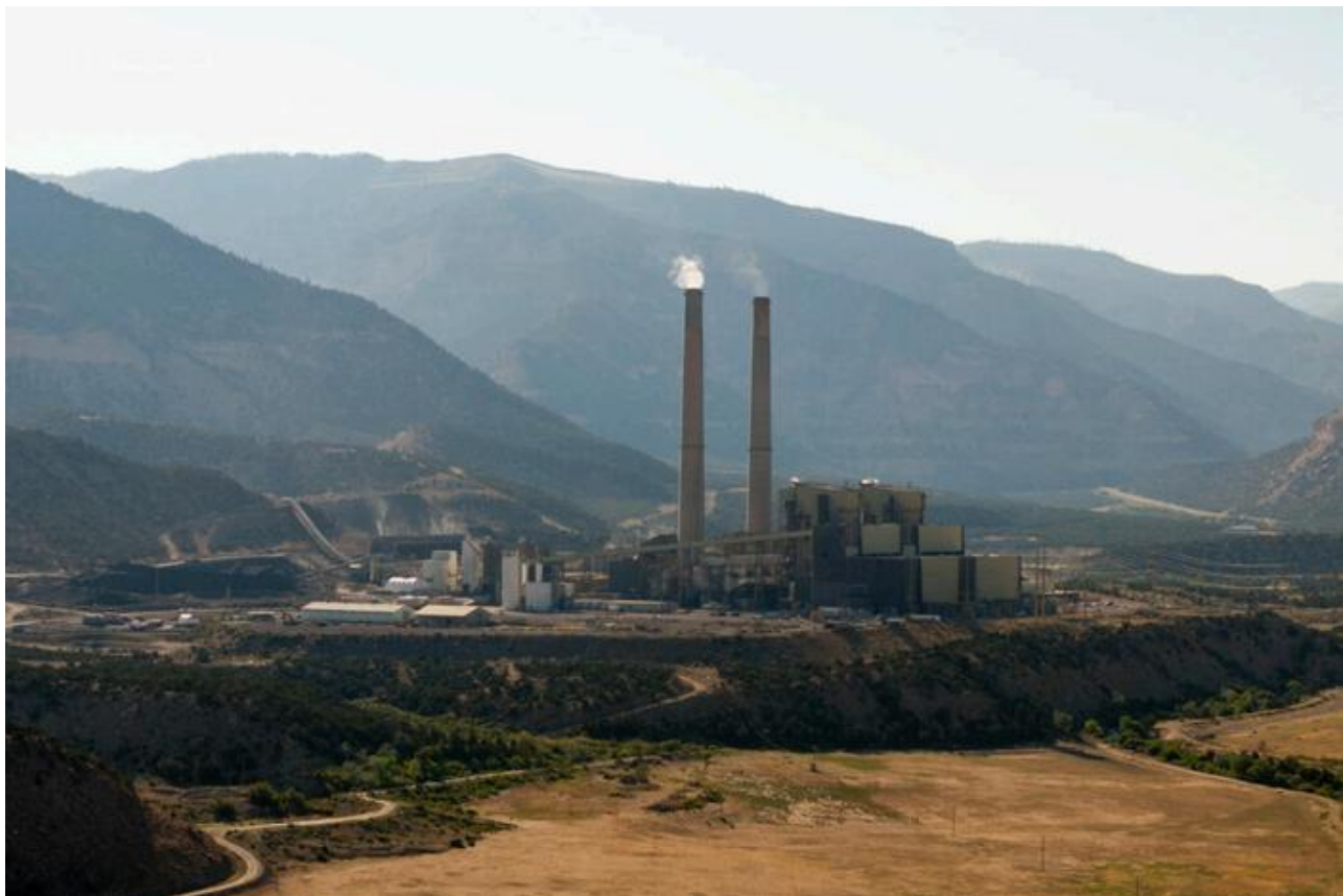
The Huntington coal-fired power plant, operated by PacifiCorp, is pictured in Emery County on Wednesday, July 31, 2024. (Photo by Spenser Heaps for Utah News Dispatch)
