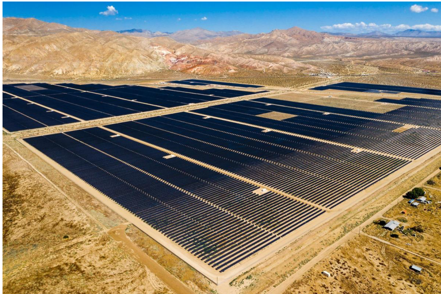
Sprinkbok 3 Power Plant, Kern County, CA
