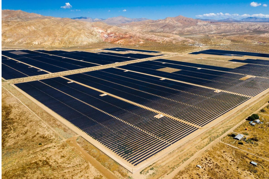
Sprinkbok 3 Power Plant, Kern County, CA
