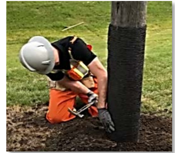
Installing Pole Wraps
