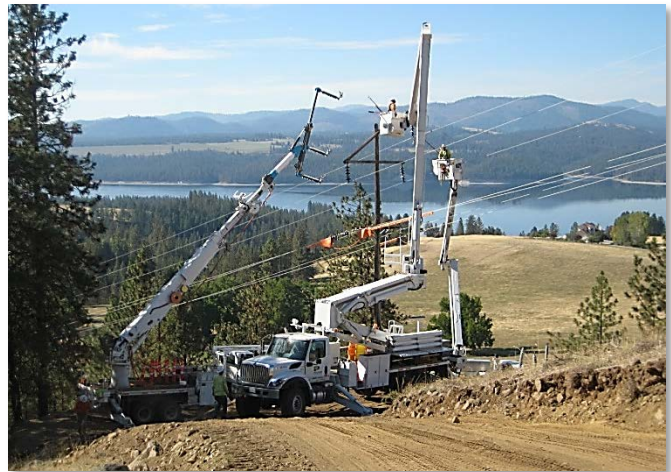
Figure 29. Addy-Gifford Steel Pole Replacement Work
