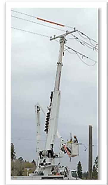
Figure 13. Grid Hardening Work
