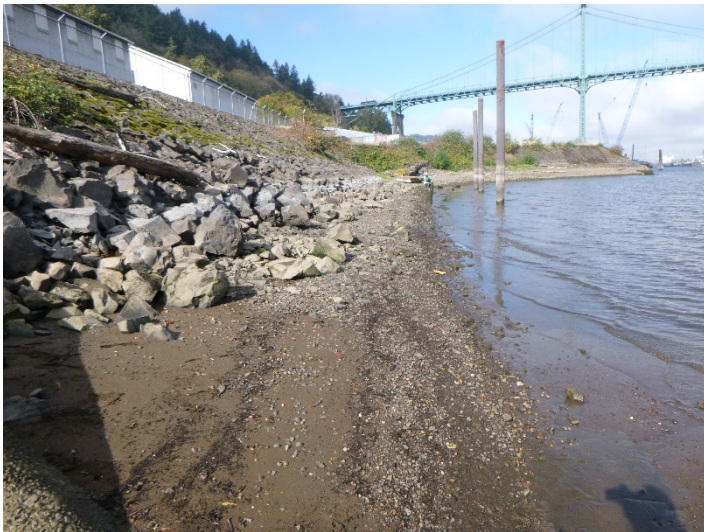
P17: South Central Portion of Project Area, From Shoreline, Looking Northeast
