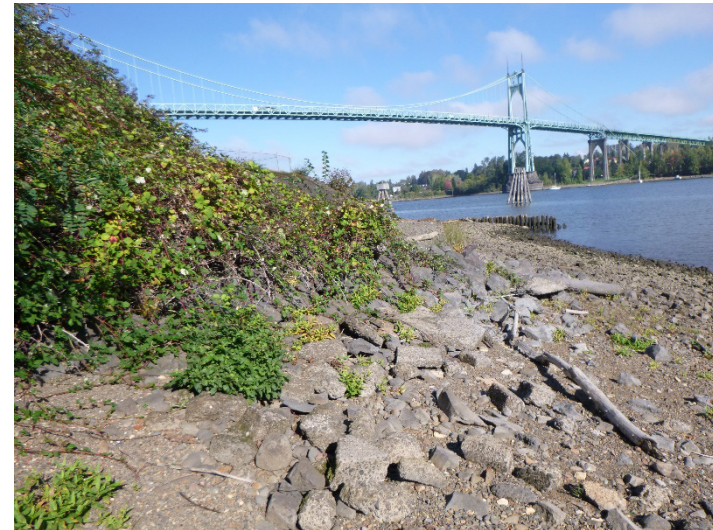
P12: North Central Portion of Project Area, Toe of Slope, Looking North
