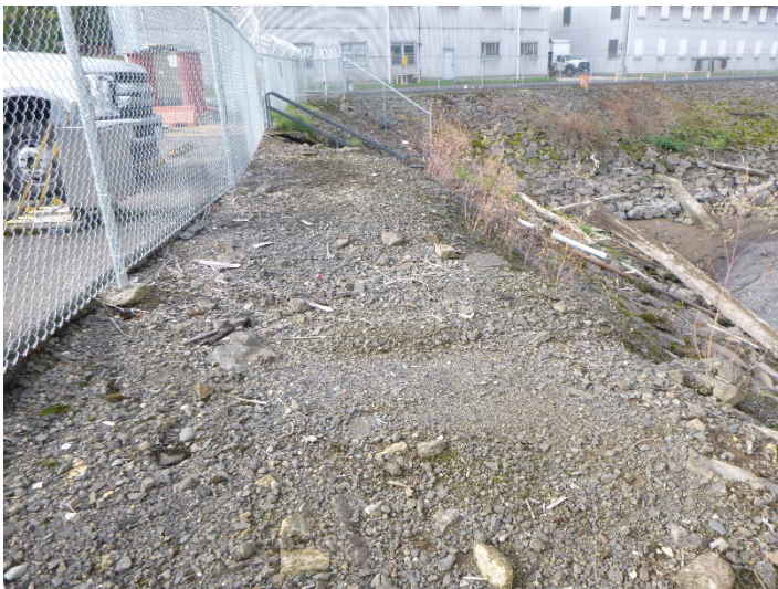
P19: Southern Portion of Project Area, Top of Shoreline, Looking West
