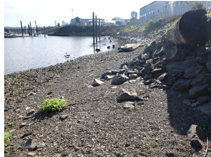
P14: North Central Portion of Project Area, From Shoreline, Looking Southeast
