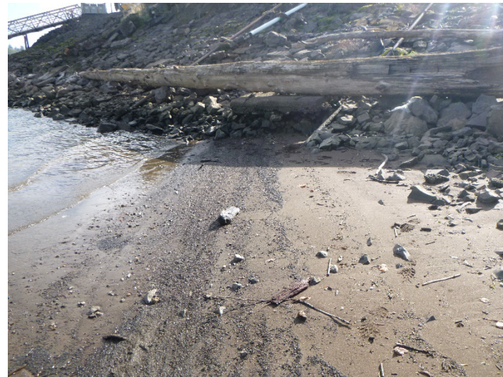
P18: South Central Portion of Project Area, From Shoreline, Looking Southeast
