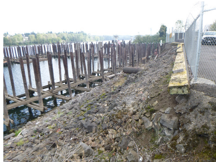
P4: South Central Portion of Project Area, Top of Shoreline, Looking Southeast
