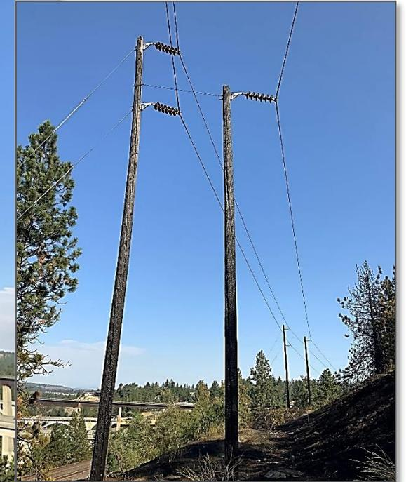
*Two of our transmission poles in Spokane were damaged by a small fire started by a passing train.*
