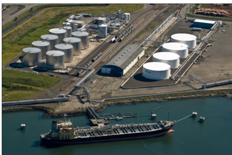
Terminal 1 at the Port of Grays Harbor operates as a barge and bulk liquid terminal. Photo courtesy of the Port of Grays Harbor.
