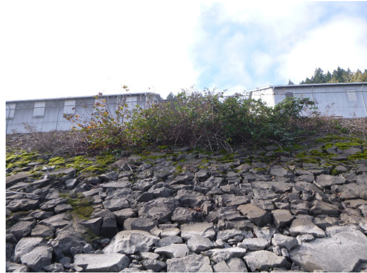
P16: Central Portion of Project Area, Toe of Slope, Looking Southwest
