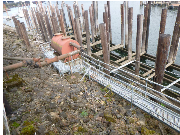
P22: Southern Portion of Project Area, Top of Shoreline, Looking North
