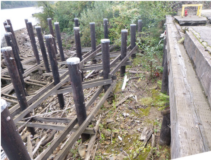
P23: Southern Portion of Project Area, Top of Shoreline, Looking Southeast
