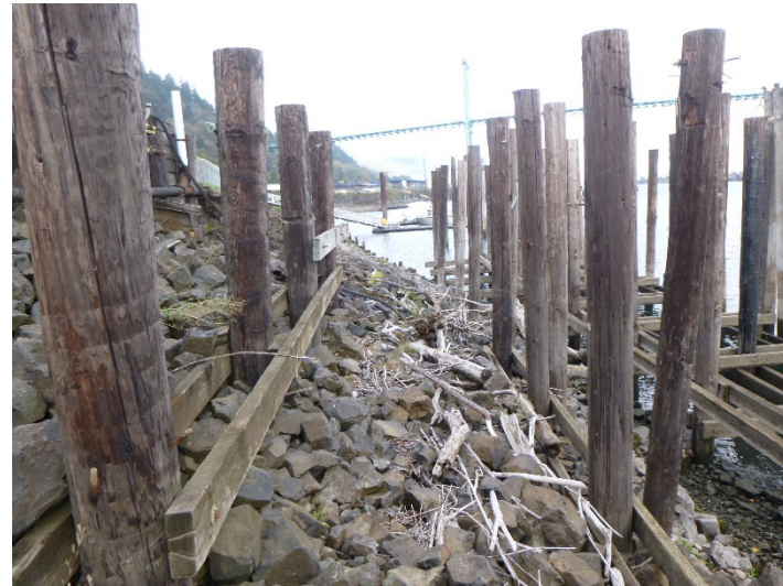
P24: Southern Portion of Project Area, Along Riprap Slope, Looking North
