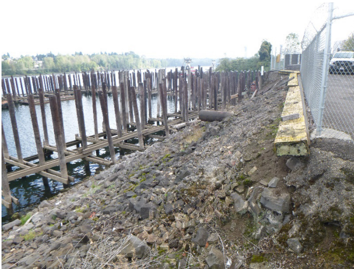
P21: Southern Portion of Project Area, Top of Shoreline, Looking Southeast
