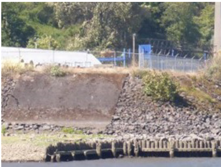
P11: North Central Portion of Project Area, From River, Looking West
