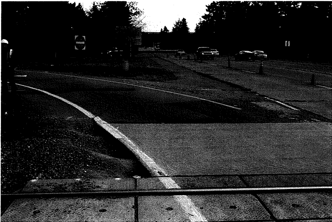
41 st Division Drive looking south
