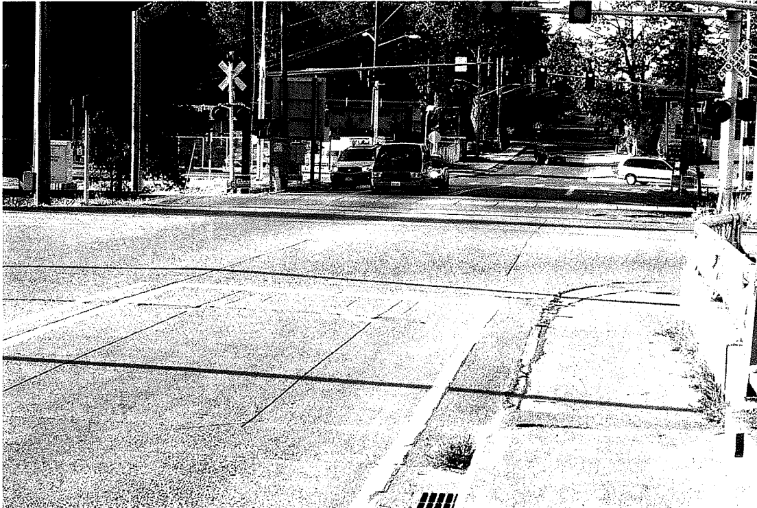
Berkeley Street SW looking north (from freeway overpass)
