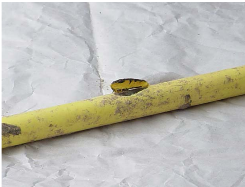
Photo 1: Photo of typical coating holiday attributed to "damaged during removal"
