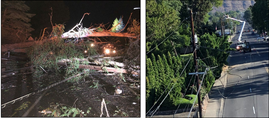
Figure 1. Photos of damaged equipment from downed tree.
