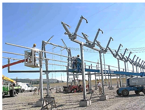
Constructing Boulder Substation
