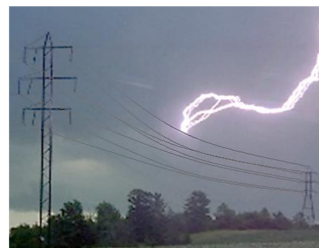
Lightning striking a shield wire
