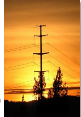
Transmission-only line of two circuits with three phases/conductors each on the bottom and a shield wire on top (no underbuild)
