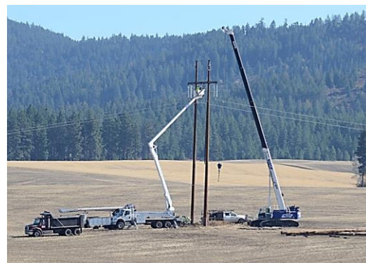
Avista rebuilding the Benewah-Moscow 230 kV line across the Palouse
