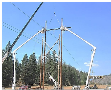
Hot Springs – Noxon #2: Replacing old wood structures with steel
