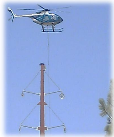
Placing conductor using a helicopter (above) and by hand (right)
