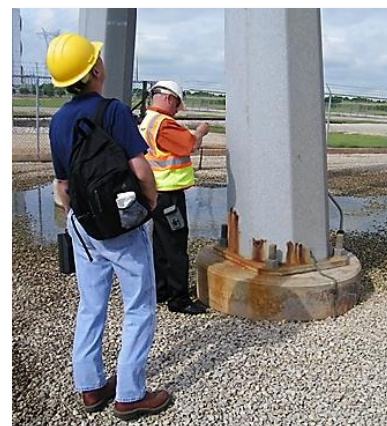
Steel Pole & Foundation Inspection
