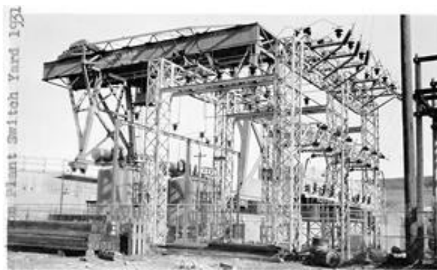
Lewiston Switch Yard in 1931
