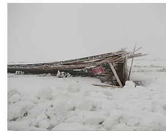
Snow & ice loading in Reardon breaks conductor and shatters a pole
