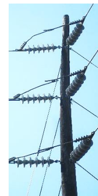
Above: String of Glass Insulators Left: Strain Insulators on a corner pole
