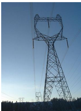
BPA's Bell-Coulee 500 kV line, built to help relieve congestion between Grand Coulee Dam and Spokane to the West Coast. (Avista's 230 line visible on the left.)
