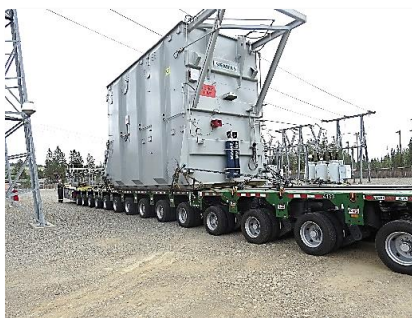
Above: Westside #1 230/115 kV Transformer Left: Westside #2 Transformer
