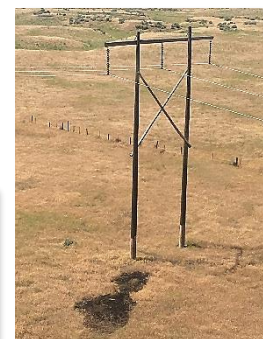
Above: Aerial inspection spots a lightning strike next to a pole
