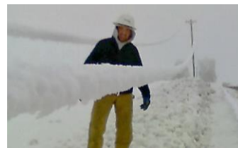
Snow/Ice loading causes a line to sag in Spokane
