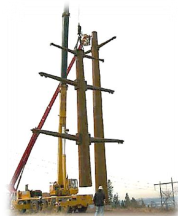
Constructing the Palouse 230 kV line
