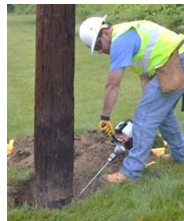
Wood Pole Inspection
