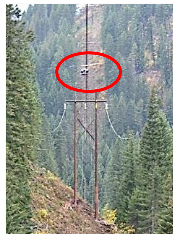
Helicopter flies the Pine Creek – Burke Thompson line
