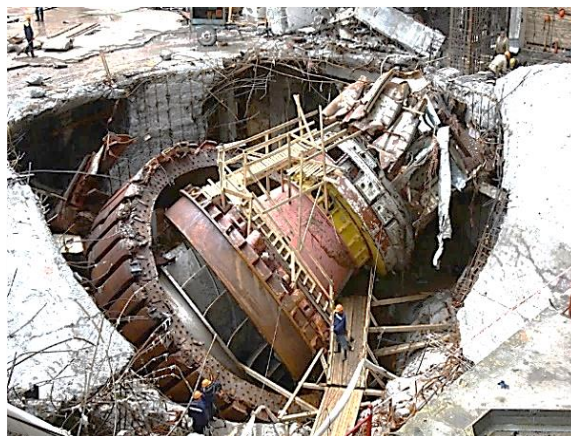
Turbine failure in Australia when it went out of synchronization with the grid and its protection equipment failed
