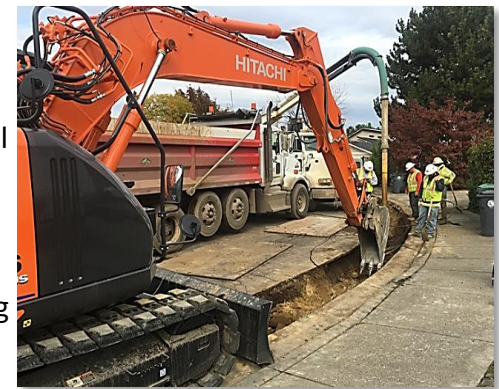
Open trenching is often required to install new gas pipeline
