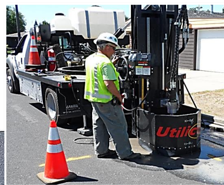
Above: Using keyhole technology to minimize road damage
