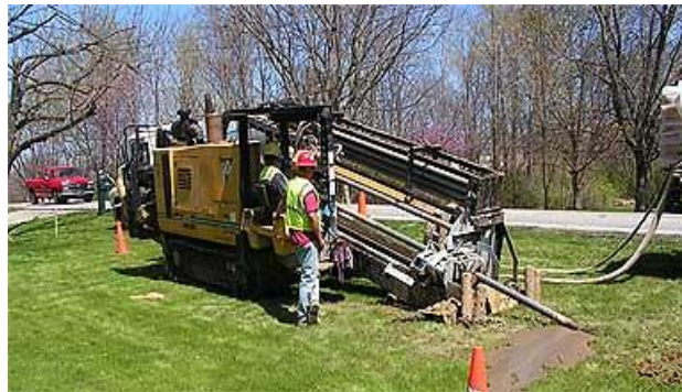
A horizontal drilling machine being used to replace main pipe
