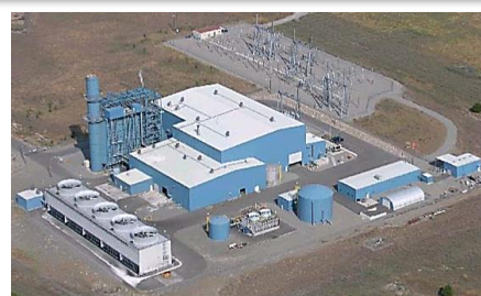
Right: Lancaster Natural Gas Plant
