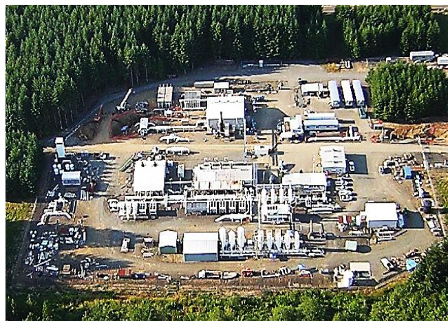
Jackson Prairie Underground Storage Facility
