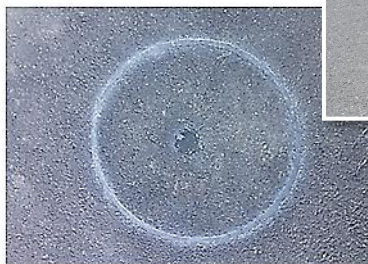
Left: The replaced keyhole core showing minimal road damage
