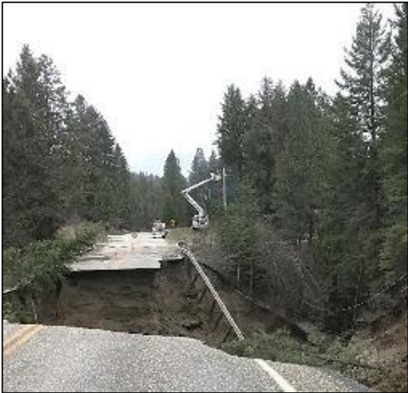
Above: Restoring power after a washout. Right: Wind storm damage
