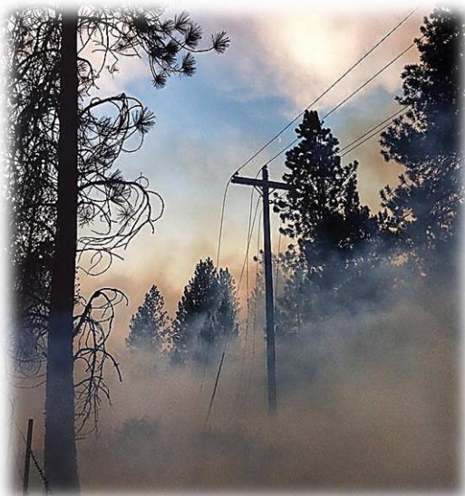
Distribution Line destroyed by wildfire
