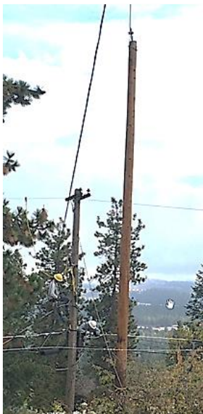
New pole being set with a crane
