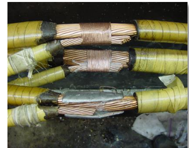
The complex process of filling paper insulated lead cable with lead to create a solid splice is a specialty of this crew
