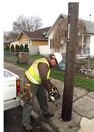
Avista Pole Inspection
