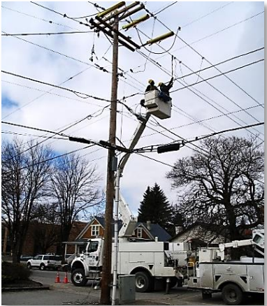
Spokane Linemen deal with the complexity of multiple foreign utilities located on their poles
