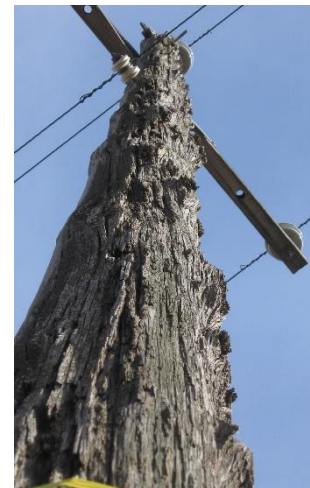
Some of the Avista Distribution poles installed in the 1920's and 1930's are still in service today... and it shows!
