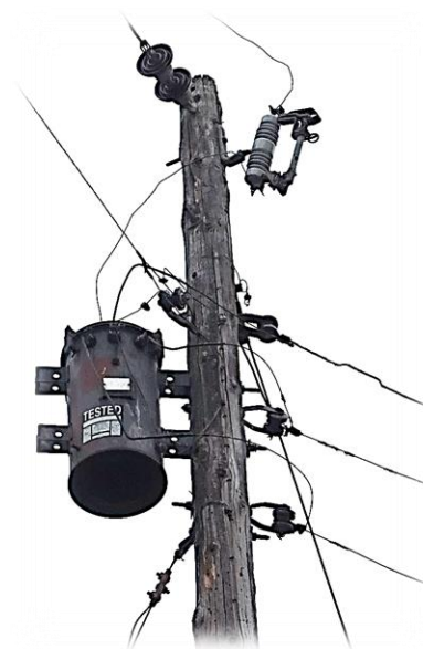
Old equipment increases reliability risk
