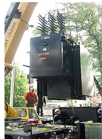
Placing a Pad Mount Transformer
