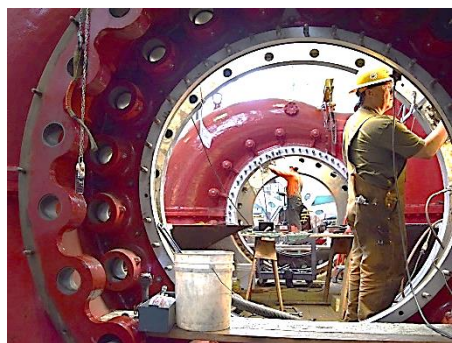
Maintaining a hydro unit
