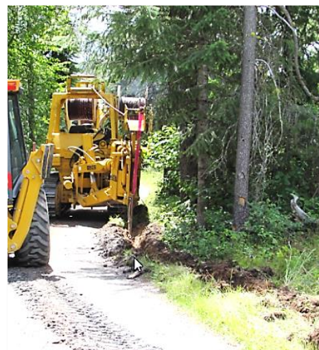
Installing underground cable
