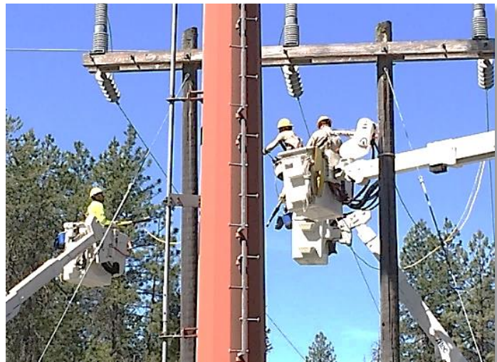
Deer Park Crew repairing transmission
