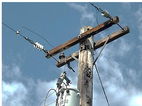
Above: Fire damaged pole Below: Broken crossarm
