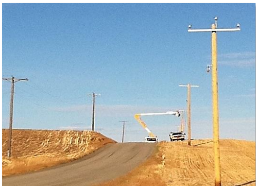
Old line on the left, new on the right
