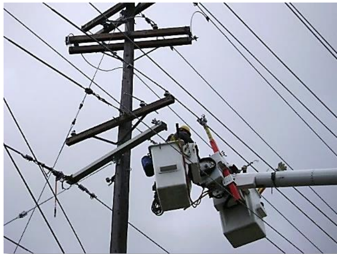
Overhead distribution work
