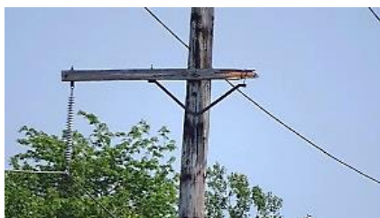
Above: Fire damaged pole Below: Broken crossarm
