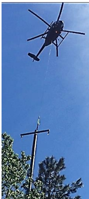
Using a helicopter to reach inaccessible areas
