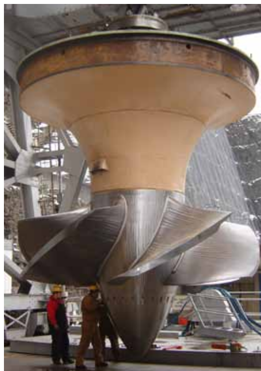
Noxon Rapids turbine upgrade
