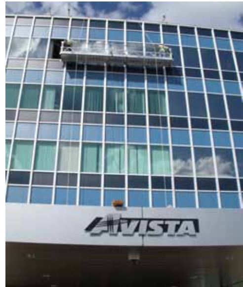
Energy efficient window replacement at Avista's headquarters in Spokane, Washington
