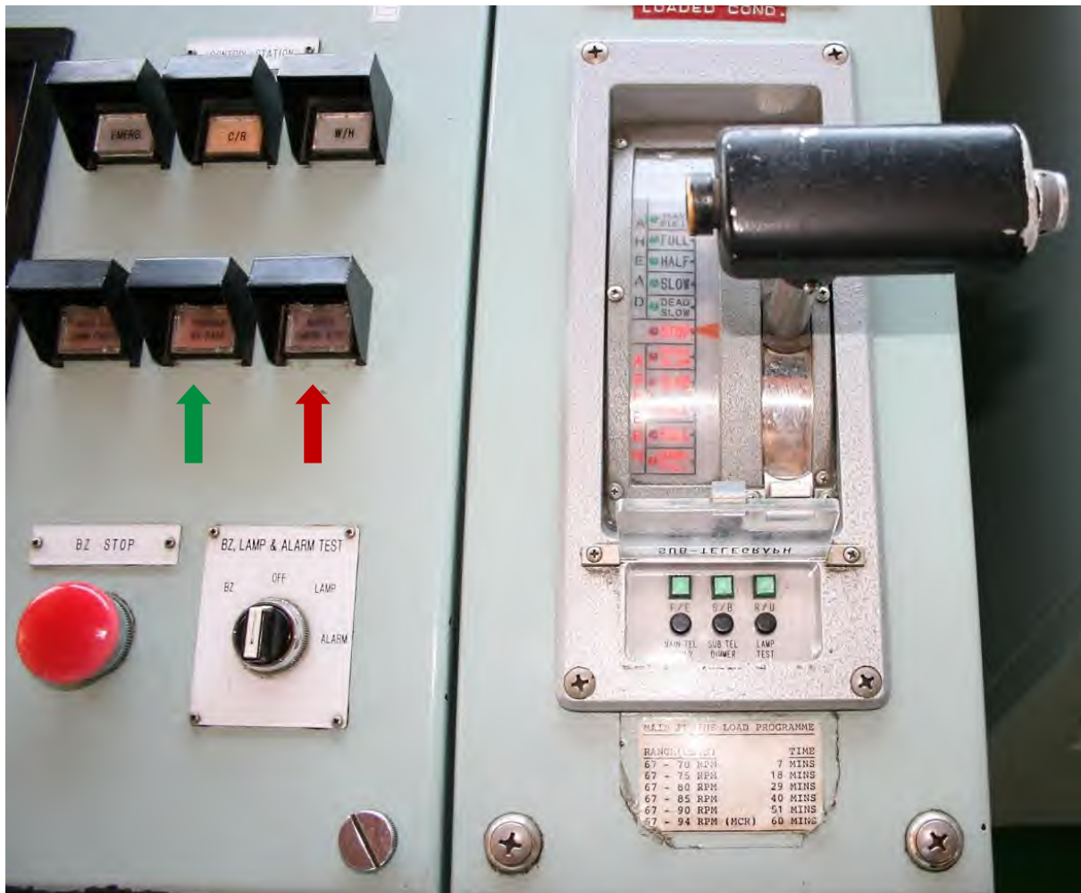
Figure 8. Section of the engine control console on the Eagle Otome . Activating the navigational full ahead required pushing the button marked with a green arrow. However, the master inadvertently pushed the "manual emergency stop" button, marked with a red arrow. (The arrows were added to this image; they are not featured on the actual engine control console.)
