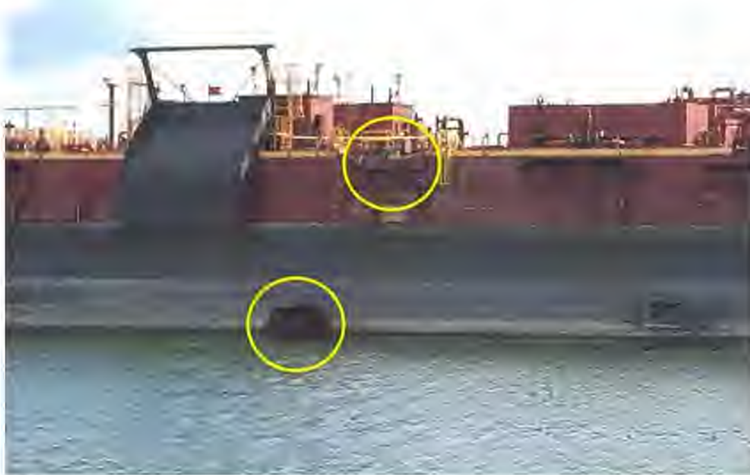
Damage to OSG 243 , port side. Yellow circles identify, at top, cantilever deck damaged by Yochow 's bow rake and, at bottom, side shell at waterline in no. 5P ballast tank penetrated by bulk carrier's bulbous bow.
